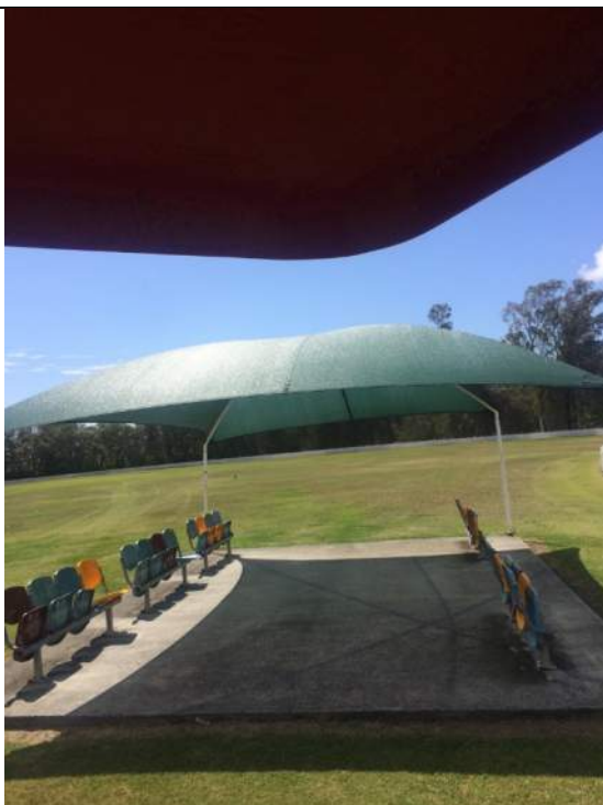
New shade structure on Wayne Broad Oval
